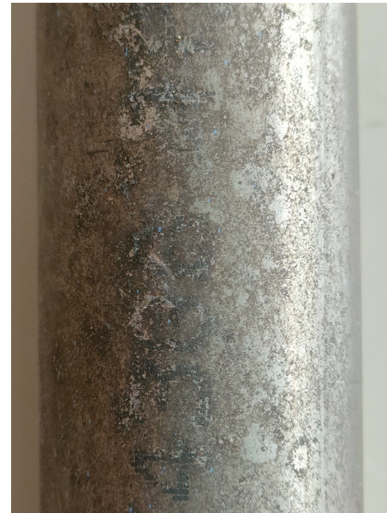
Steel pipe: rough, partially rusted
